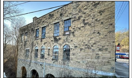
WPA BUILDING 337 MAIN STREET BEATTYVILLE, LEE COUNTY, KENTUCKY
